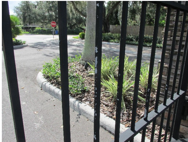
Deteriorating finishes evident
