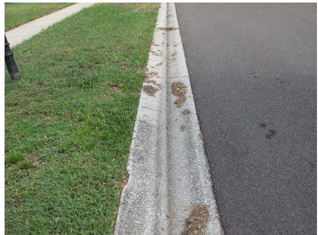
Concrete curb and gutter
