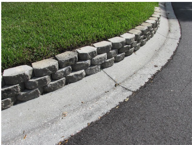
Retaining wall at entrance of community
