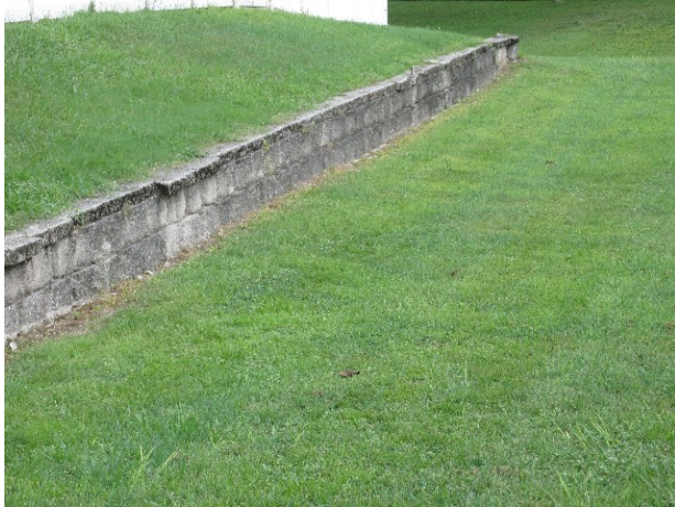
Retaining wall at pond
