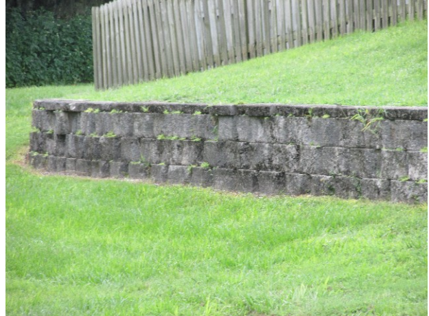
Retaining wall at pond
