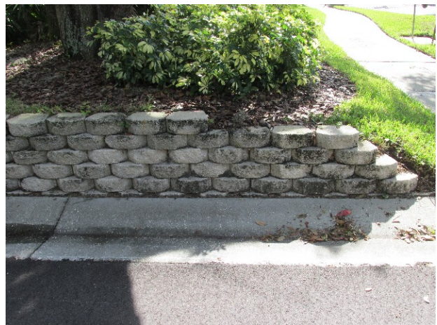
Masonry retaining wall
