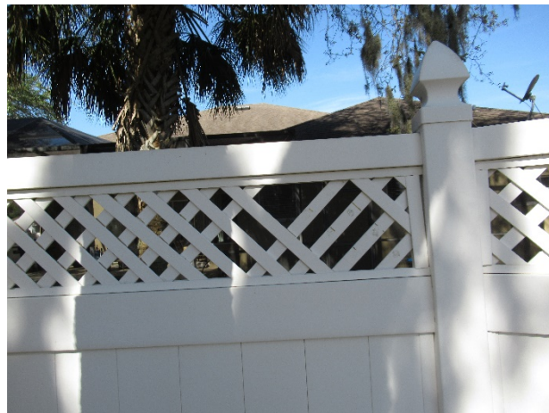
Vinyl fence with damage
