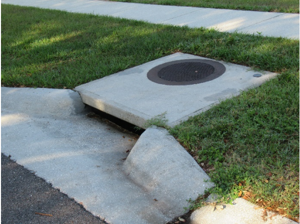
Typical catch basin
