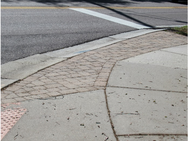
Masonry pavers at the entrance
