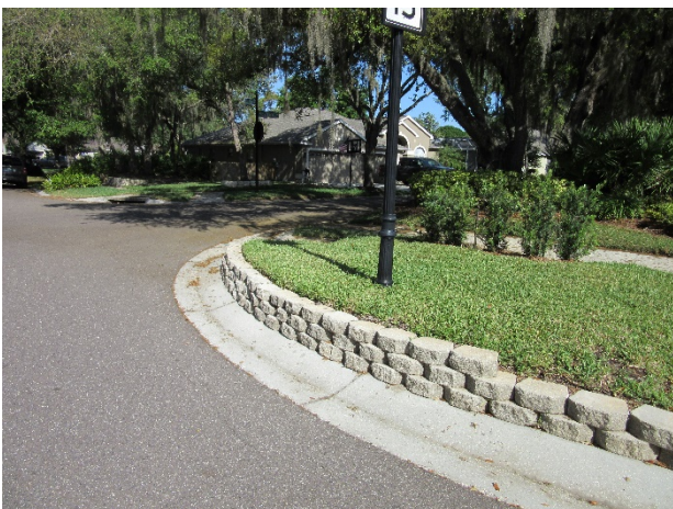
Retaining wall at 10738 Moss Island Drive
