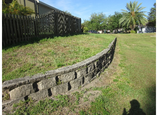
Retaining wall at 11111 Bridgecreek Drive
