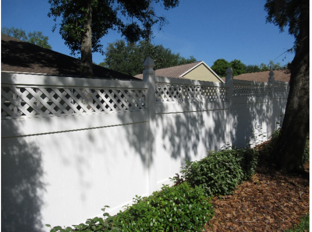
Vinyl fence overview
