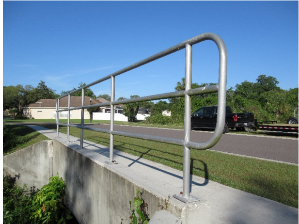
Railing above the box culvert on Moss Island Drive
