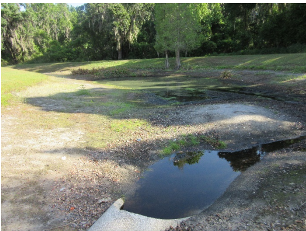
Bridgecreek Drive pond overview
