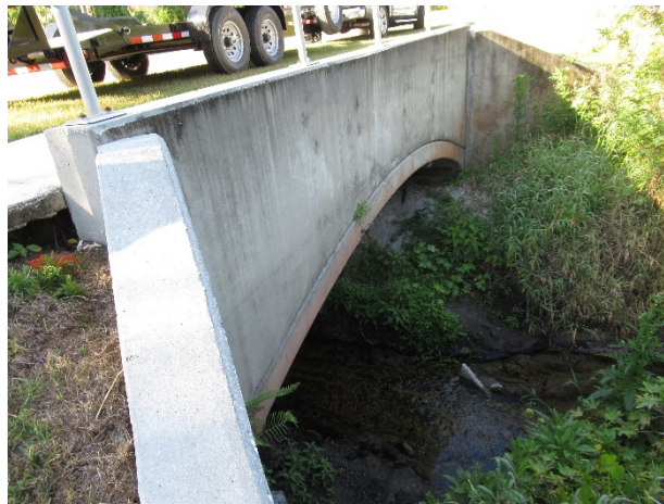
Box Culvert on Moss Island Drive
