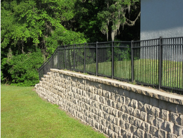
Retaining wall at Moss Island Drive overview
