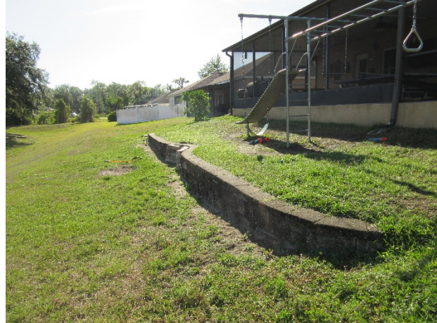
Retaining wall on South side of 11144 Bridgecreek Drive
