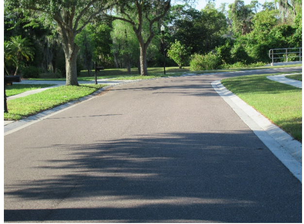
Asphalt pavement overview
