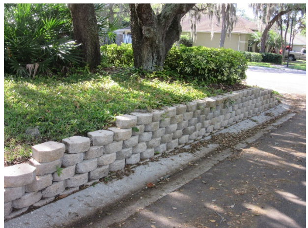
Retaining wall at 10738 Moss Island Drive
