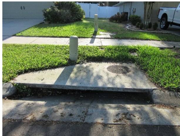
Typical catch basin
