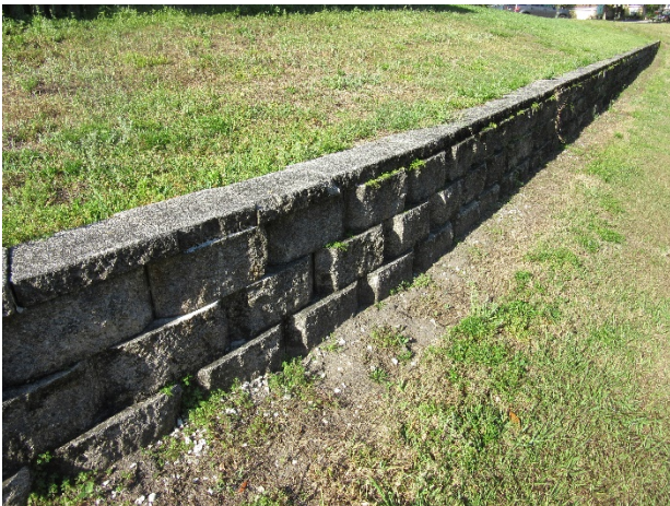
Retaining wall at 11107 Bridgecreek Drive
