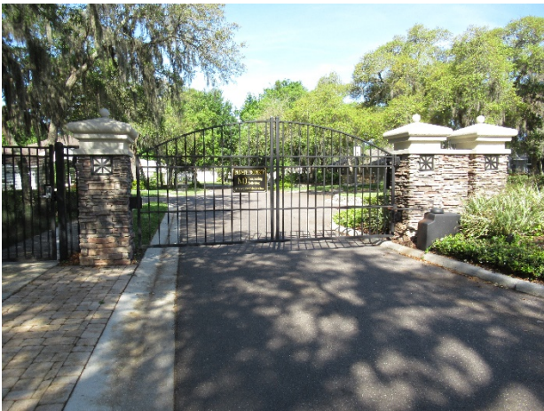
Masonry columns at the gate entry
