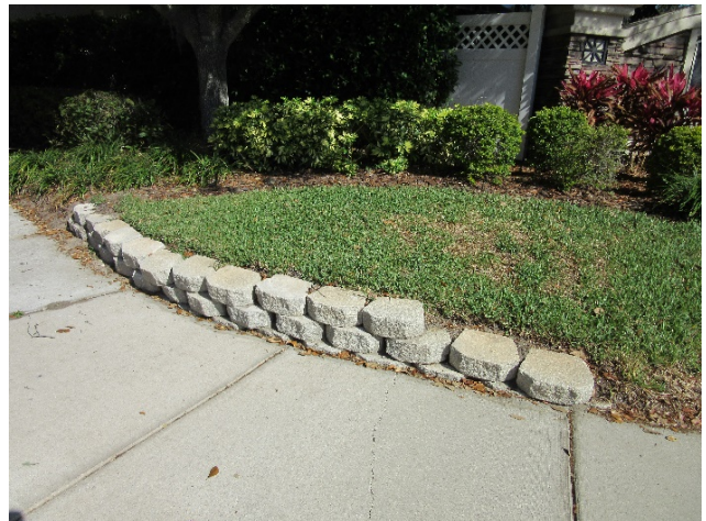
Retaining wall at the front entrance
