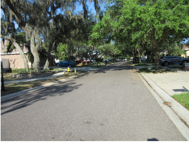
Asphalt pavement overview
